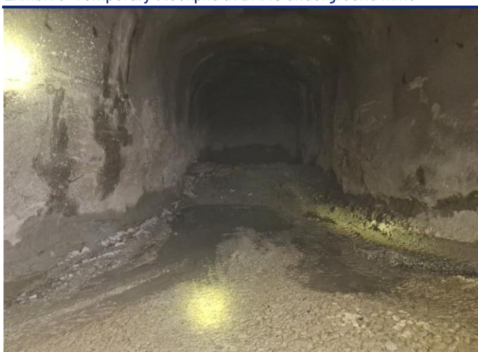
Exhibit 5. Temporary stockpile at BRMS underground mine
