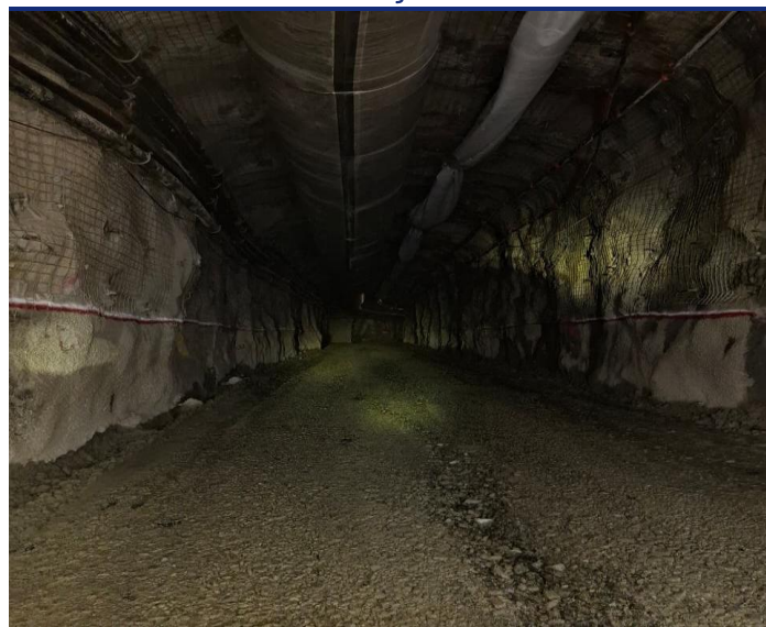
Exhibit 4. tunnel inside the underground mine
