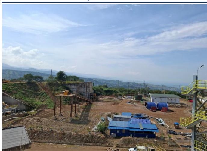
Exhibit 11. BRMS CIL 1 already dismantled
