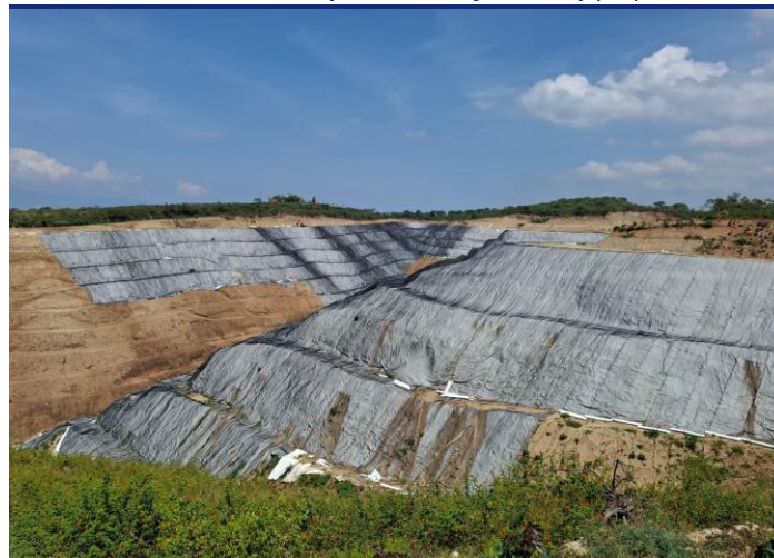
Exhibit 14. BRMS second dry stack tailings, already prepared
