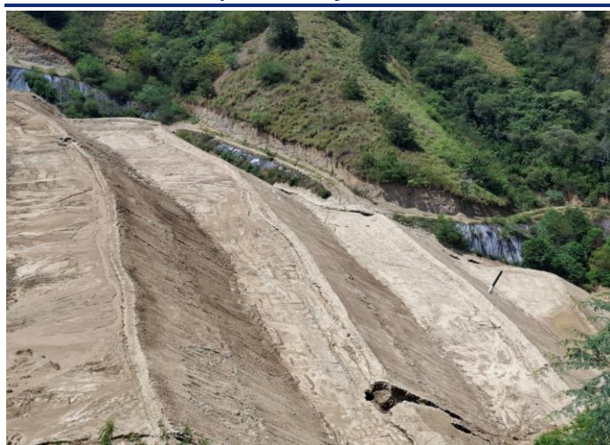
Exhibit 13. BRMS first dry stack tailings
